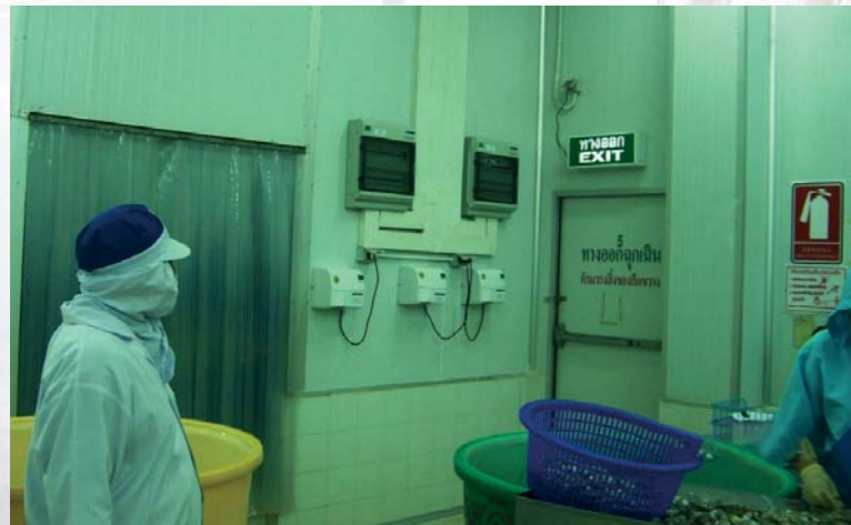
Hensel KV Small-type distribution boards in a frozen food company in Thailand
