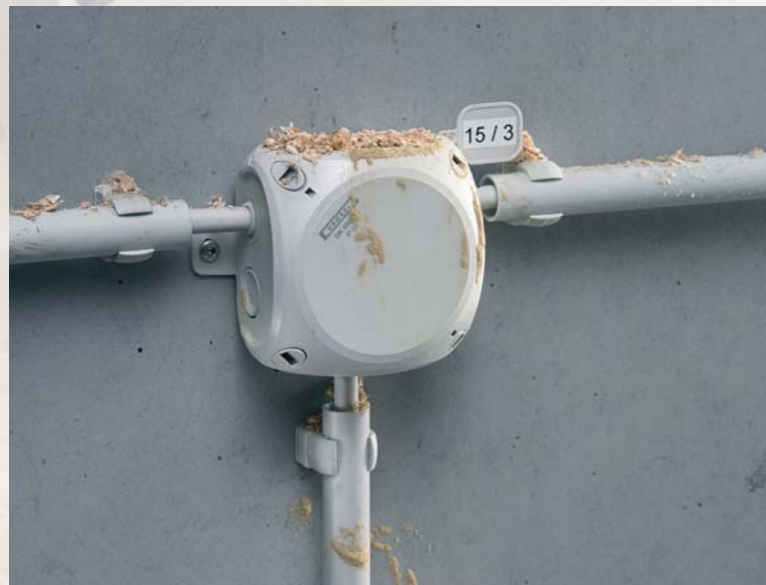
The Hensel cable junction box is dustproof (IP 66).
