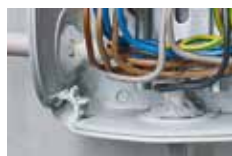
Cable retention via retention rings for cables
