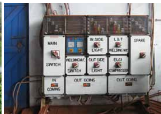
■ Power distribution board installed at a maintenance workshop of an iron ore mine
