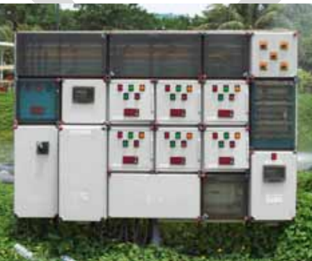
■ Outdoor distribution board installed at the lawns of a luxury hotel.
